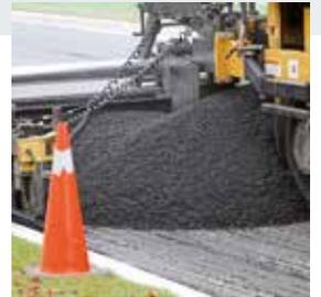
Recycled asphalt pavement
