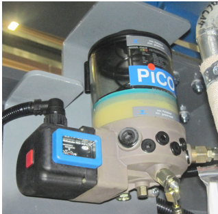
Fig. 51: Central lubrication system
