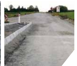
Reused for road subbase
